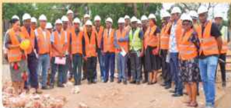
UCCMVC, Prof. Anagye (center) reminds the consultant and contractor to adhere to schedules and standards.
